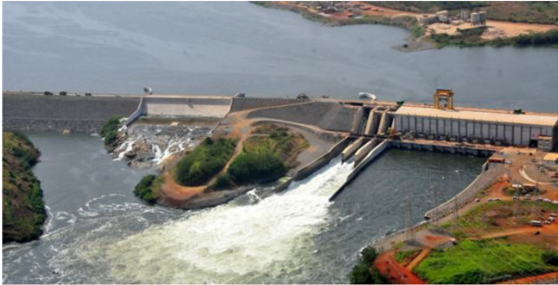
The 250 MW Bujagali Hydro Project on River Nile
